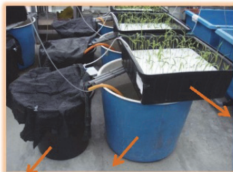
Sludge tank fish tank hydroponic tank
